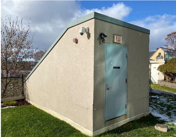
North-west stairwell structure incomplete.
