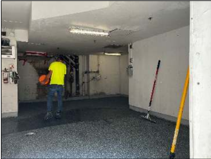
Waterproofing of the Garbage Room
