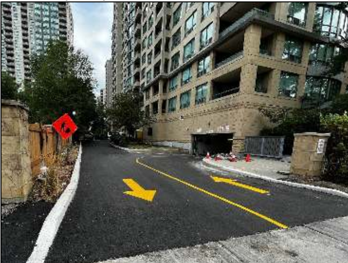
Asphalt pavement installation
