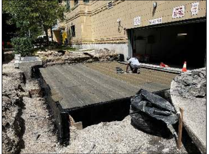
Replacement of hot-applied waterproofing at the parking garage entrance
