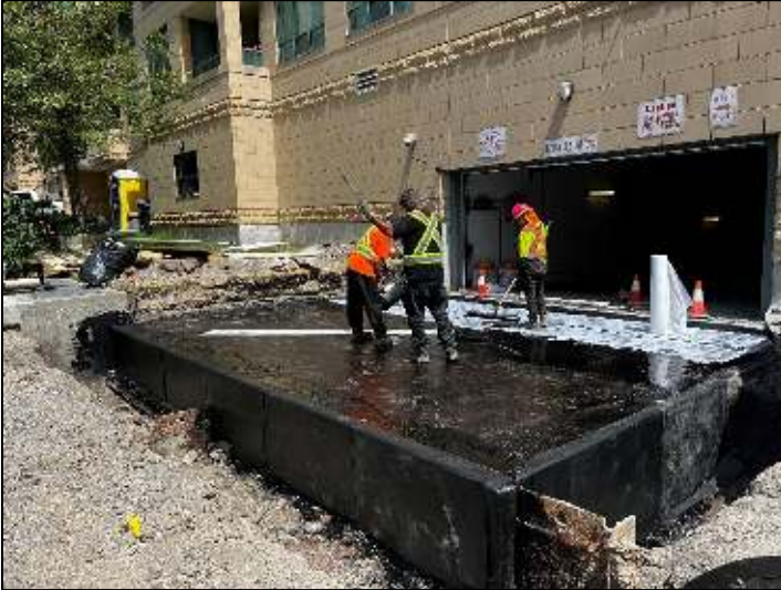
Replacement of hot-applied waterproofing at the parking garage entrance
