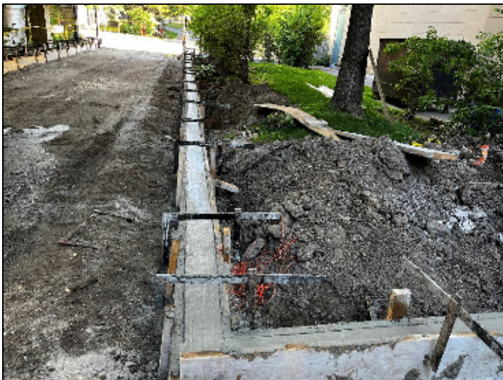
Installation of new concrete curbs
