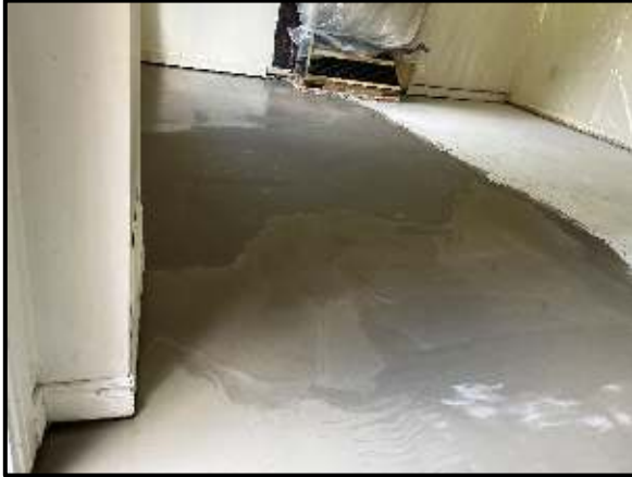
Installation of New Self-Levelling Cementitious Underlayment
