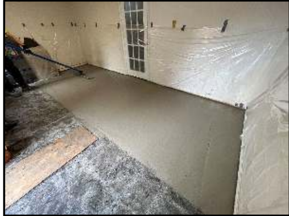
Local Replacement of On-Grade Floor Slab
