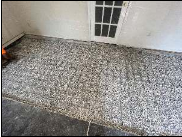
Removal of On-Grade Concrete Floor Slab
