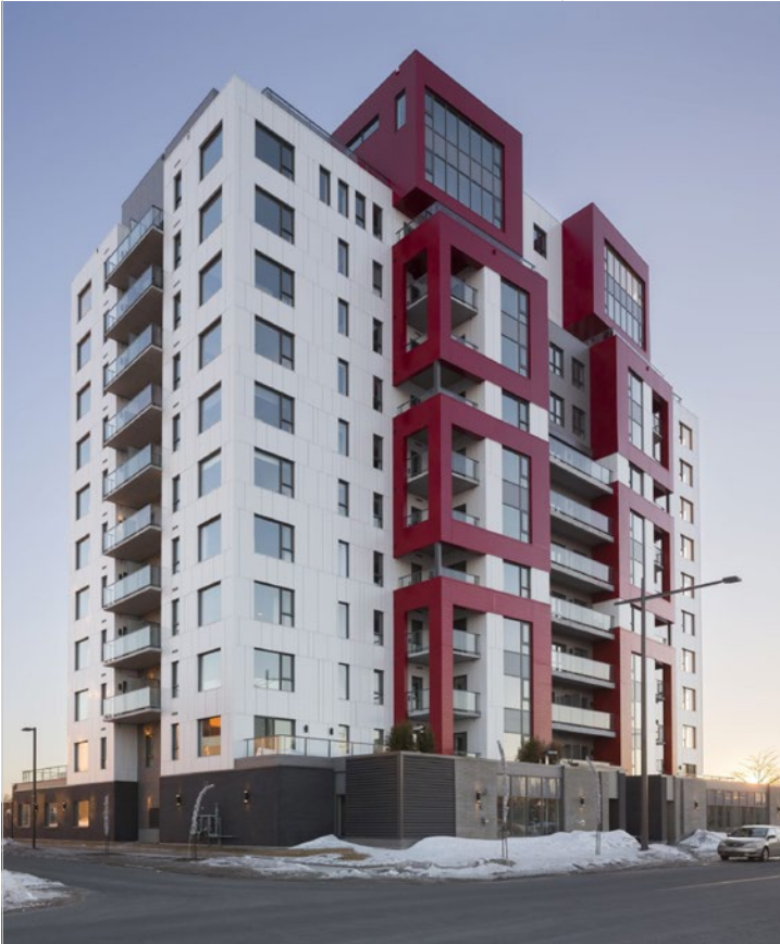
It took only four months, from December 2016 to April 2017, to erect the wooden structure of Quebec City's Origine: a 13 storey high, remarkable landmark and tallest wood building in eastern North America.
