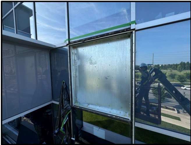
Removal of spandrel panels
