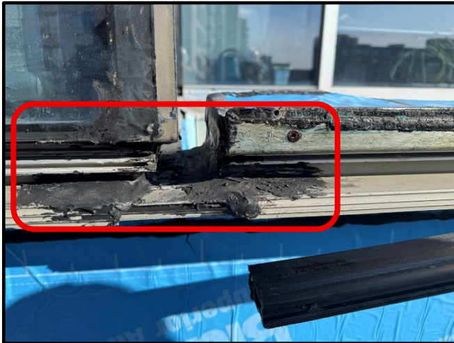
Installation of new interior window film
