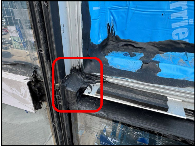
Installation of new sealants at various locations ('critical' weather seal, mullion-to-rail intersections, split mullion gaskets, parapet interfaces, etc.)
