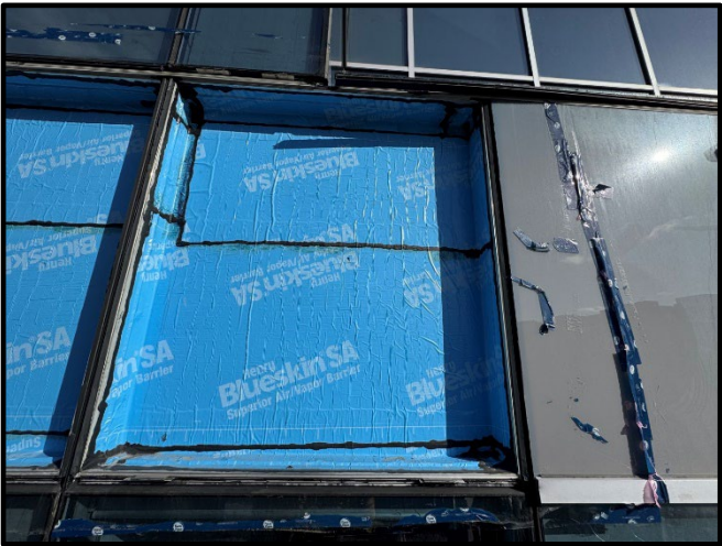
Installation of new self-adhered membrane
