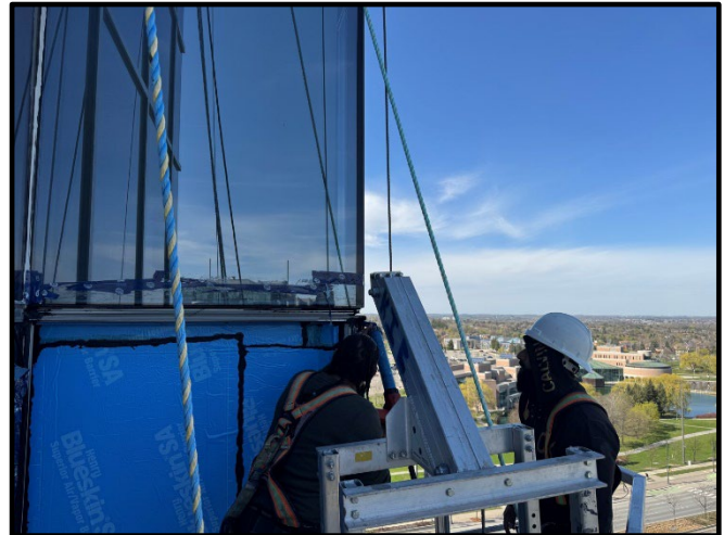
Reinstatement of spandrel panels
