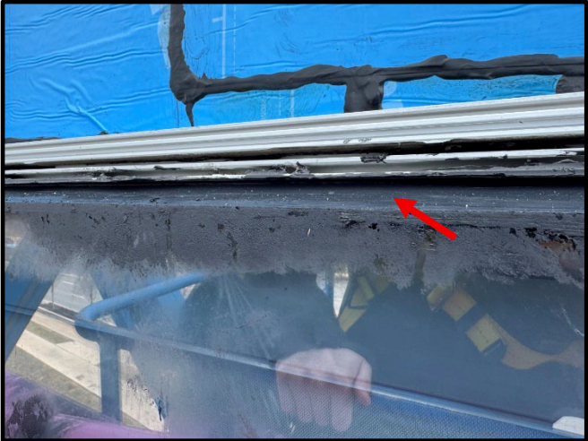
Installation of new sealants at various locations ('critical' weather seal, mullion-to-rail intersections, split mullion gaskets, parapet interfaces, etc.)
