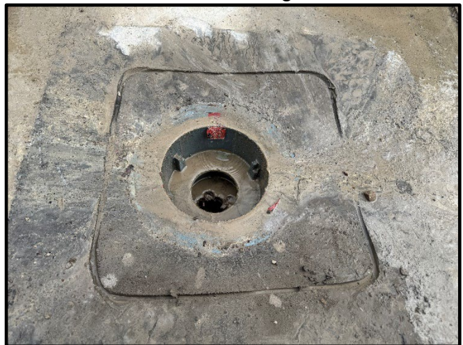
Installation of New Garage Roof Drain
