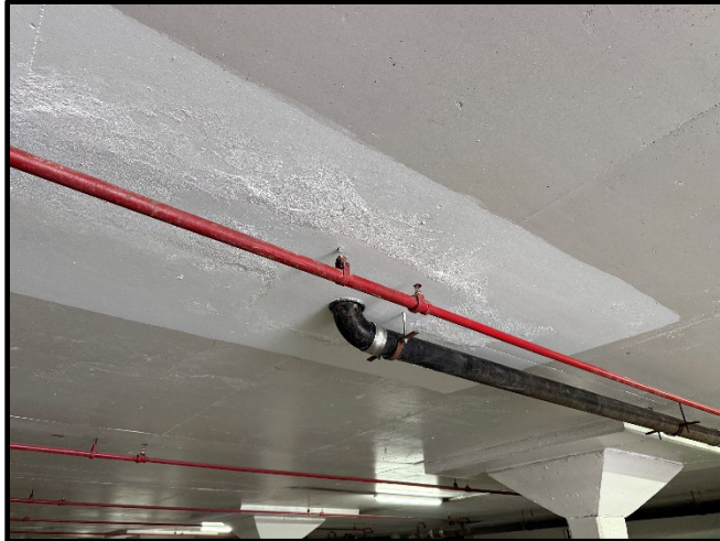
Installation of Drainpipes
