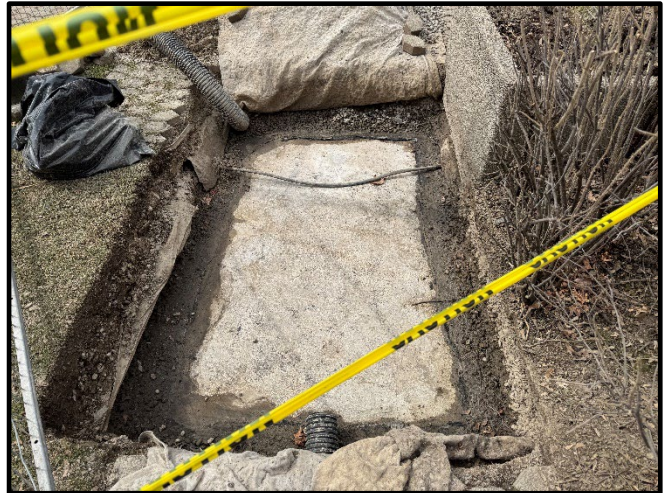
Removal of Existing Waterproofing and Surface Preparation of Concrete Slab
