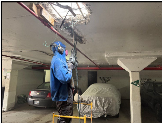
Removal of Delaminated Concrete
