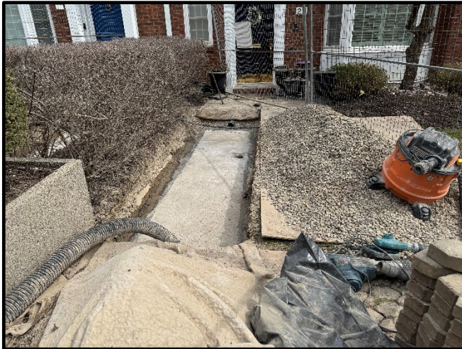
Removal of Delaminated Concrete
