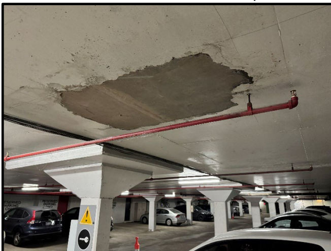
Installation of Concrete at Soffit Repair Areas
