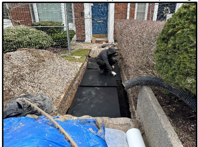
Installation of new Hot Applied Waterproofing
